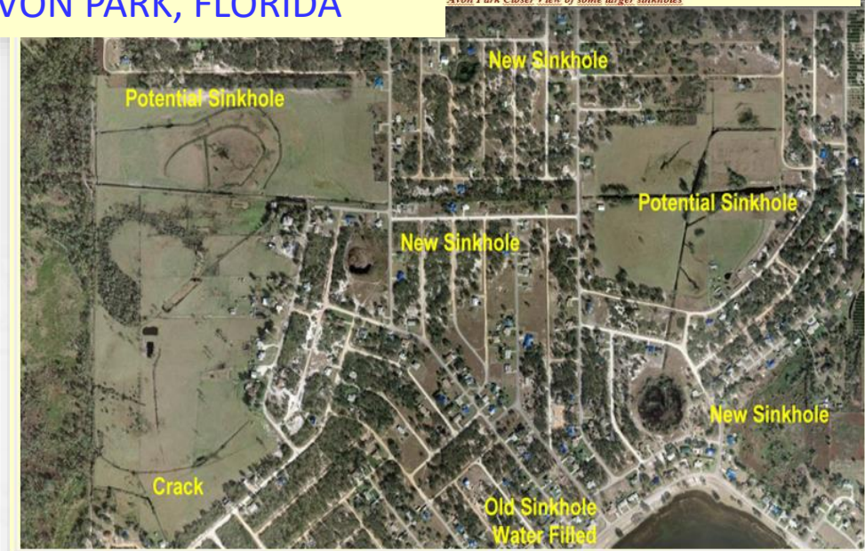
Avon Park, Northwest Corner... new sinkholes and signs of others ready to break open
